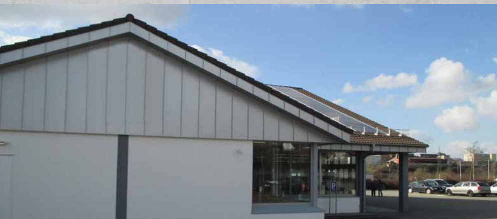
Anbau Discounter, Gemrigheim
